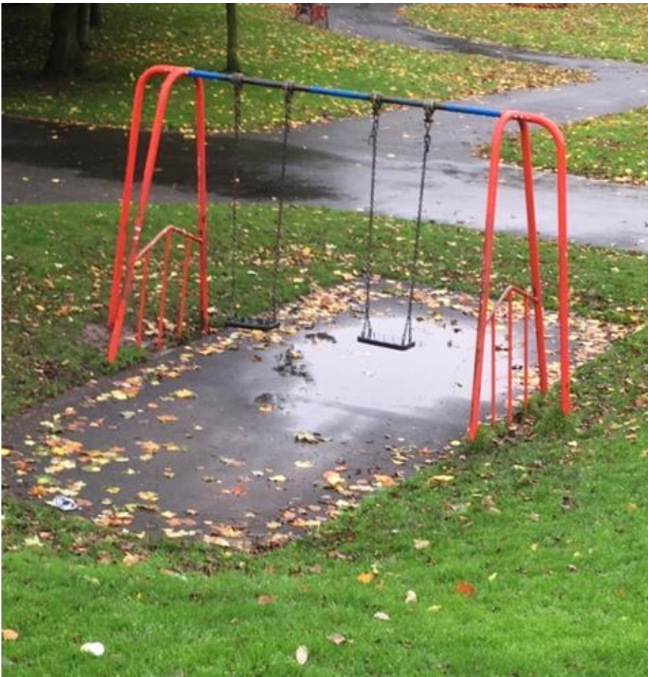
Replacement of grass matting with wetpour under double swings at Dukinfield Park £2500
